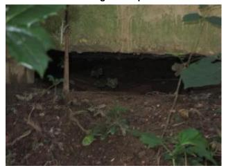
CLOSE UP OF SUB SLAB EROSION @ CARPORT #GC
