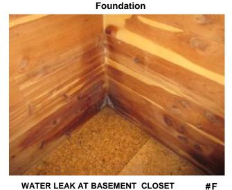
WATER LEAK AT BASEMENT CLOSET
